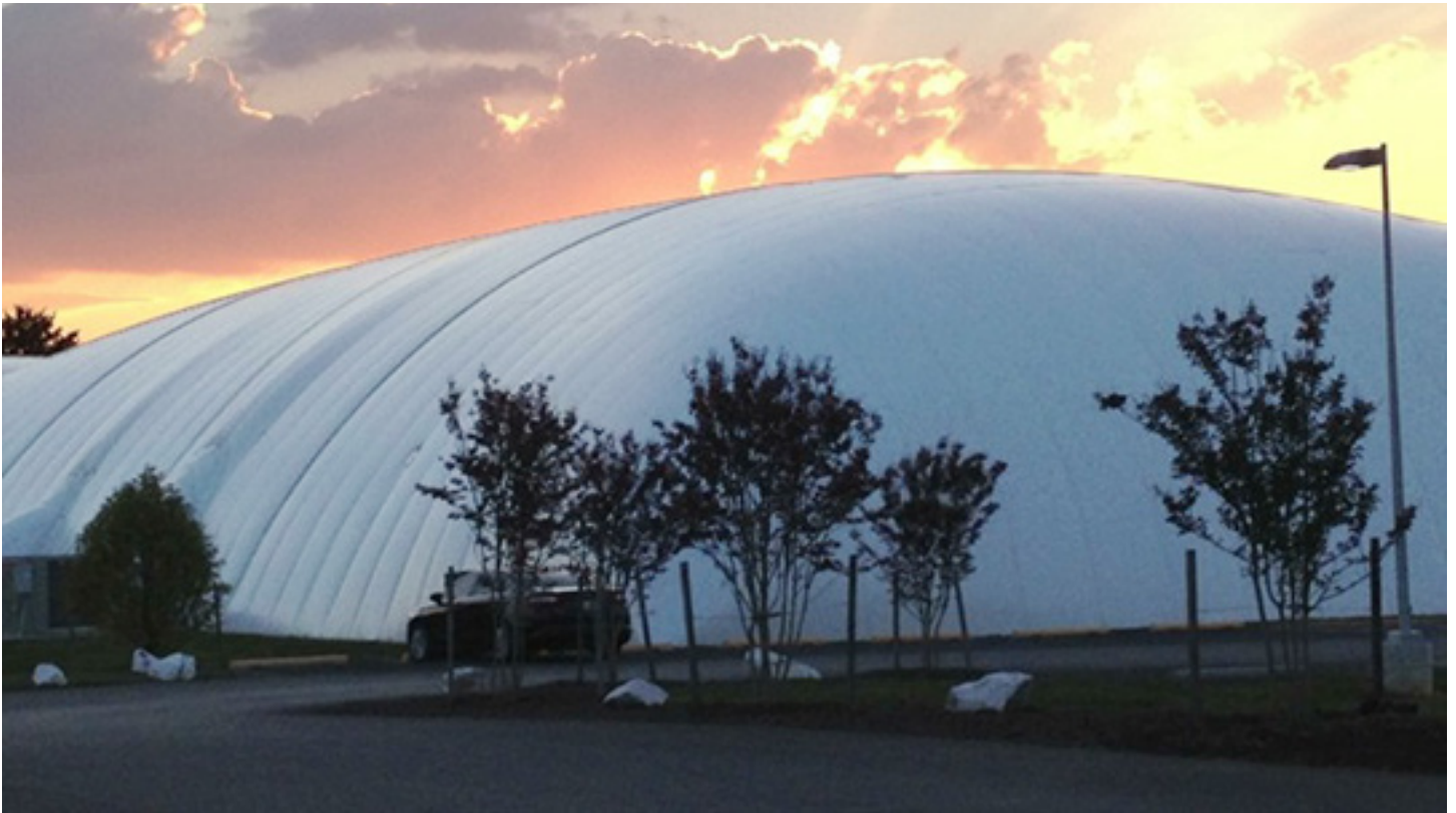
The two bubbles which house eight courts allow for play with no worries regarding inclement weather.
